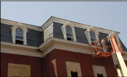
Bloch Industries installs the new dormers.
