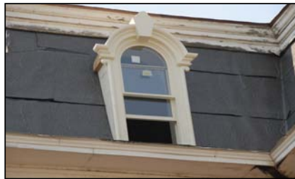
Our beautifully restored dormer windows.
