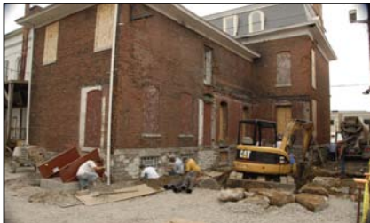
LockTight Waterproofing installs drainage and seals the basement.
